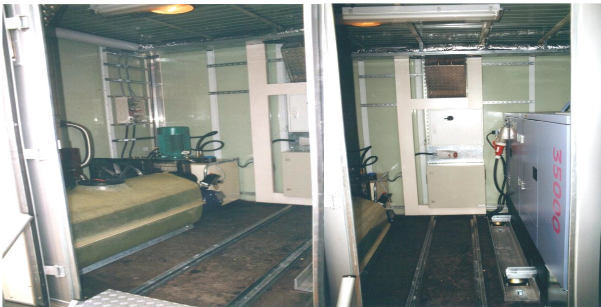
Abb. 30: Hydraulik, Kompressor, Wassertank
