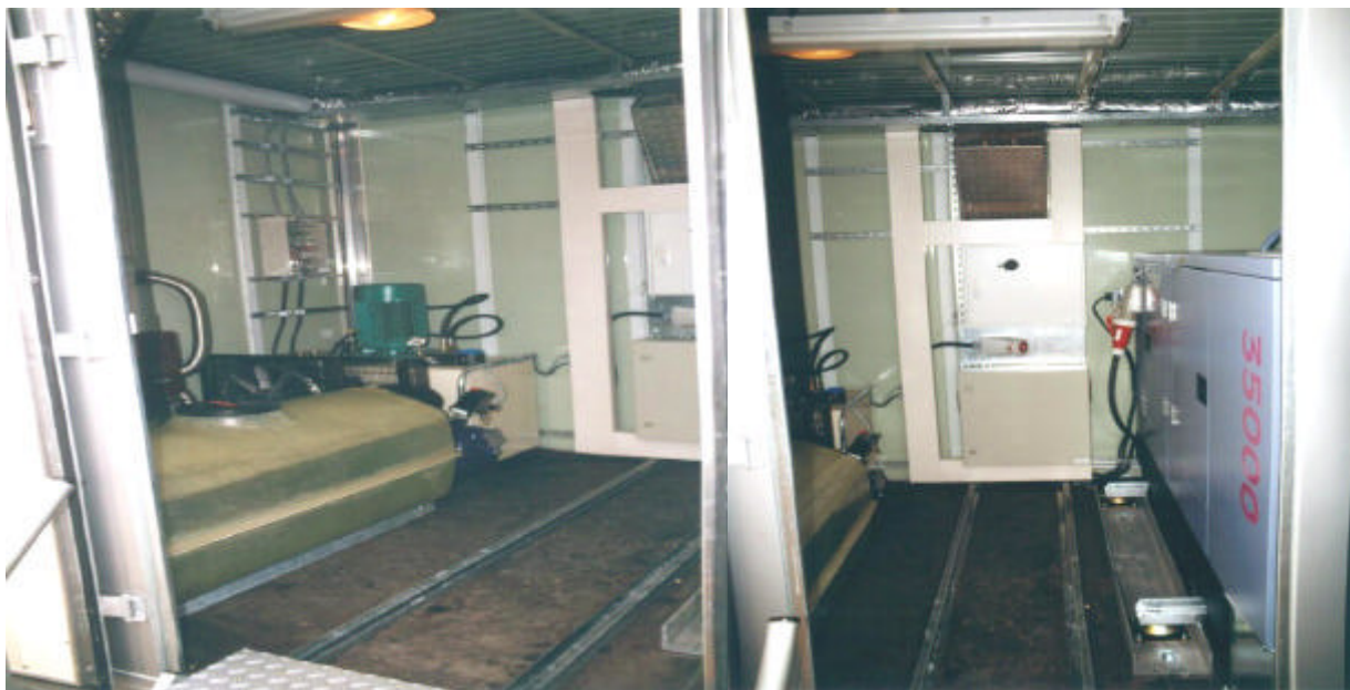
Pic. 30: Hydraulic, Compressor, Water tank
