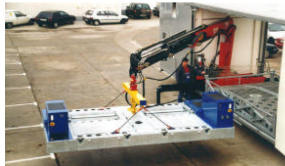
Pic 12: Positioning the test units
