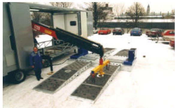
Pic. 14: Positioning of the ramps
